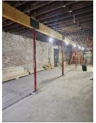
The Worthy Ambition Team has replaced the center wall with an engineered post and beam system to open the first floor to an open-concept 1,600 square foot retail space.
