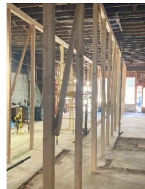
Temporary supports were designed and installed until new engineered posts and beams are placed.
