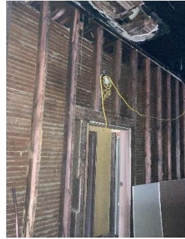
The dividing wall between two retail spaces is being removed to provide more than 1,500 square feet of retail space on the first floor.
