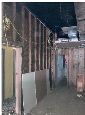
Temporary supports were designed and installed until new engineered posts and beams are placed.
